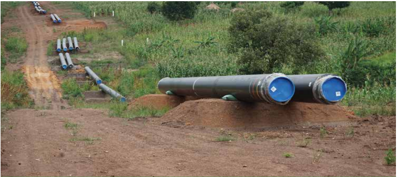
Feeder Pipelines erected and passing through farm lands in Buseruka, Hoima
